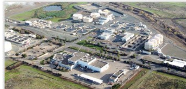
Delta Diablo Wastewater Resource Recovery Facility (Wastewater Treatment Plant + Recycled Water Facility)
