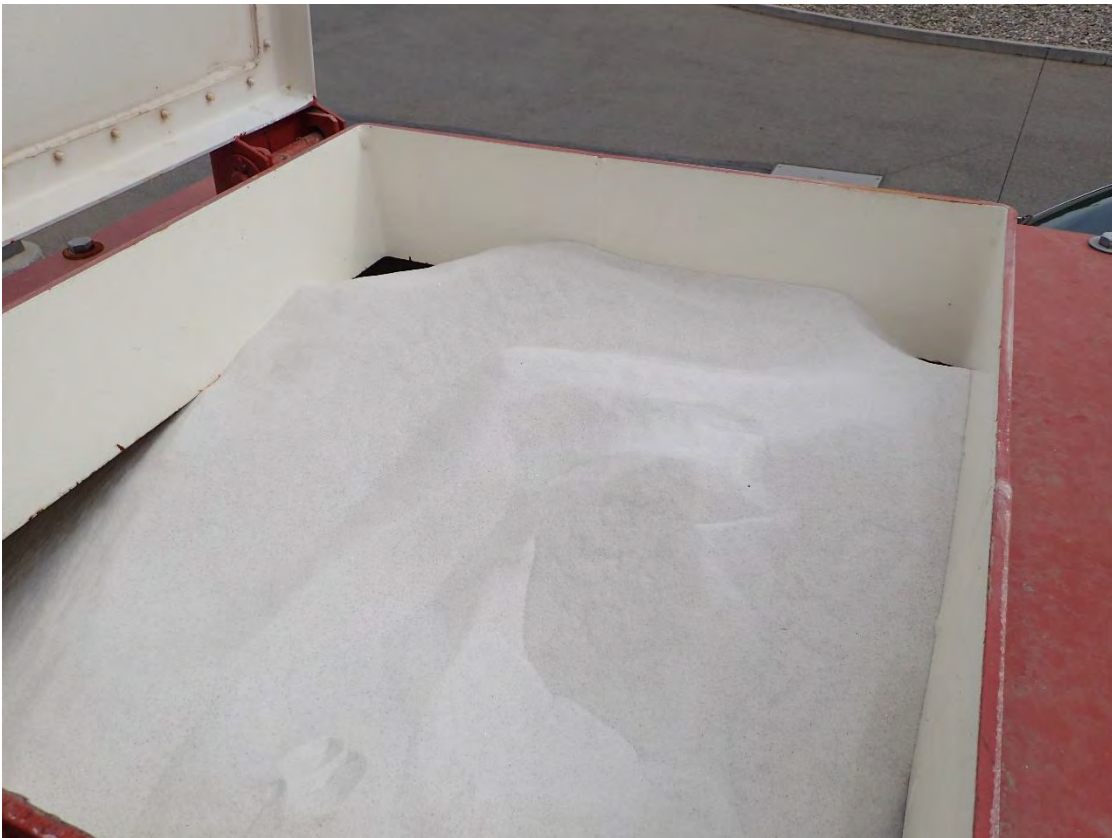
12. Sand for recycled water plant.
