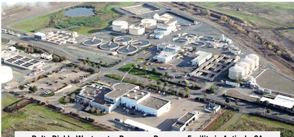
Delta Diablo Wastewater Resource Recovery Facility in Antioch, CA (includes Wastewater Treatment Plant and Recycled Water Facility)
