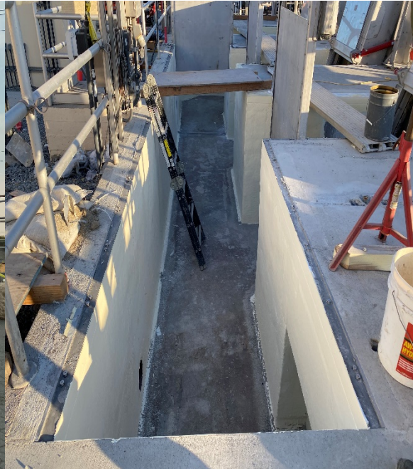
Rehabilitated headworks channels
