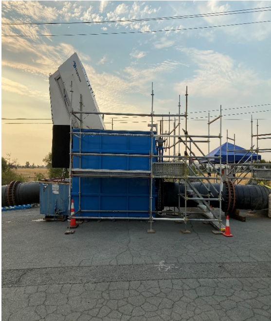
25.5 MGD temporary pumping and screening
