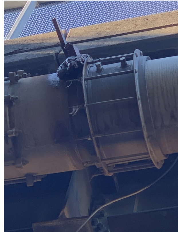
Initial temporary repair at expansion joint
