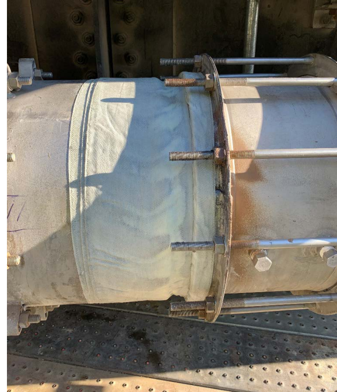
Improved temporary repairs
