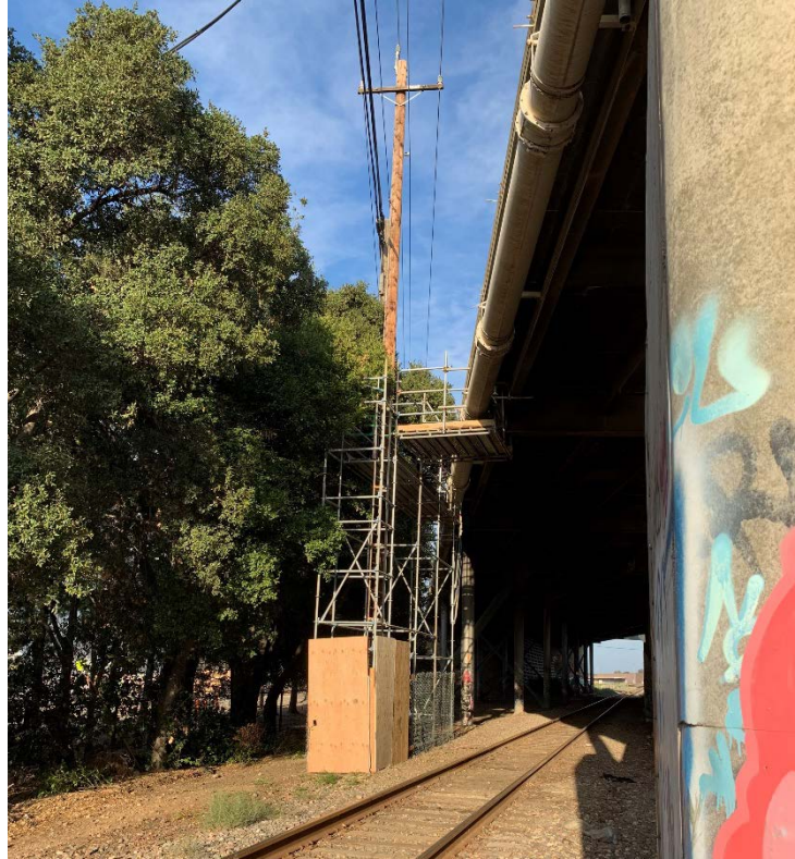
Scaffolding to access pipeline and allow train movement
