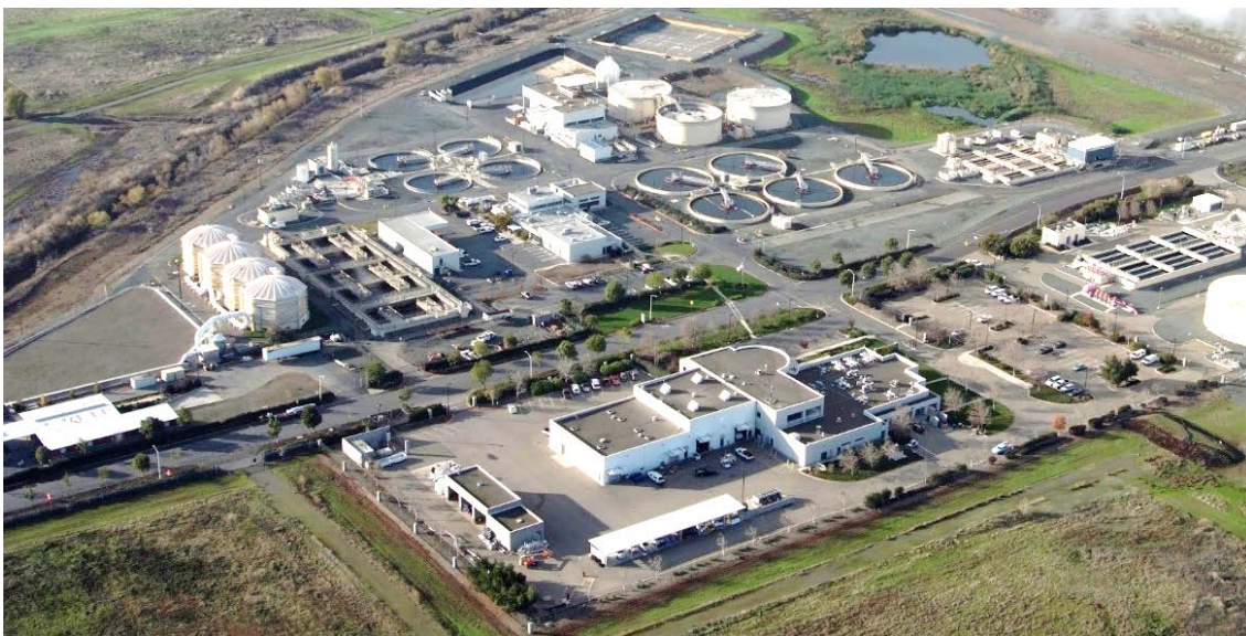
Delta Diablo Wastewater Treatment Plant in Antioch, CA
