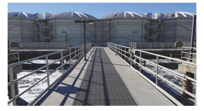
Tower Trickling Filters and Aeration Basins
