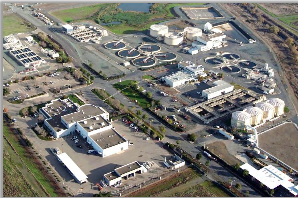
Treatment Plant and District Offices
