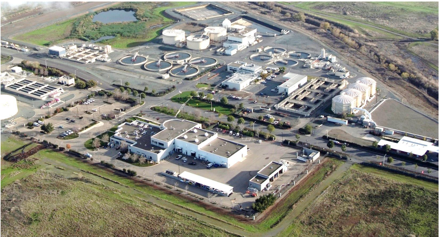
Delta Diablo Wastewater Treatment Plant in Antioch, CA
