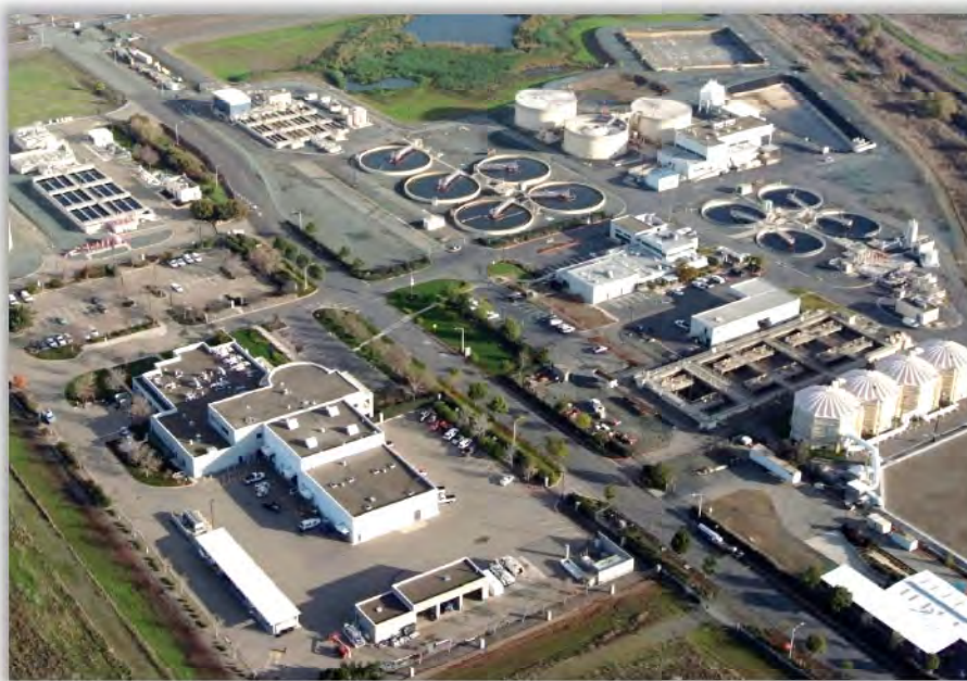
TREATMENT PLANT AND DISTRICT OFFICES
